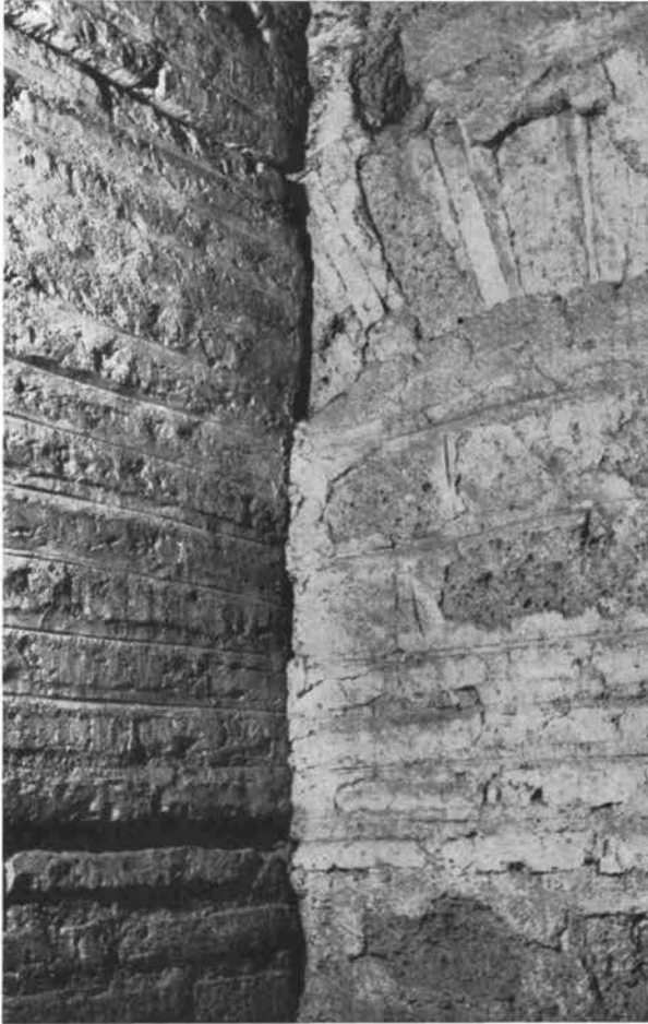
Fig. 228 — S. Maria in Cosmedin. Correspondence of the diaconia opening, the campanile (left) and the wall which seals the opening (Photo: Corbett).
